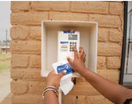
Non-technical losses, which include illegal connections, theft of equipment and vandalism, amounted to between 3 730GWh and 5 968GWh for 2014/15. Installation of split metering with protective enclosures is one of the interventions undertaken to reduce these losses
